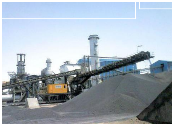
Sirjan iron ore concentrate Plant
