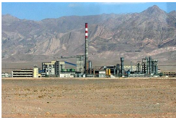
Zarand Coke Making Plant
